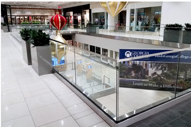
Custom stainless steel cladding forms fit over the aluminum shoe and extend below to cover the top-mounted shoe, lending a continuous look on balconies.
