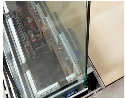
*Pressure plate system consisting of a 3/8" nylon - 1 1/4" steel - 3/8" nylon block assembly between the glass and stair stringer. A 3/8" thick nylon and 3/8" thick steel pressure plate, mimicking the same profile and cut as the stringer, finished off the exterior of the pressure plate assembly.*
