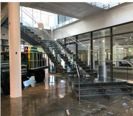
*A combined 186 linear feet of Trex Commercial Products' Point Series, glass treads and risers were used to create a clean, minimalist look for the building lobby.*
