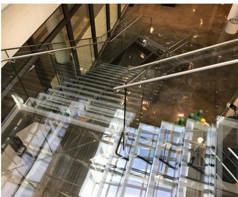
*Glass treads and risers, combined with the Trex Commercial Products' Point Series railing system, give this staircase a seamless, barely there appearance.*
