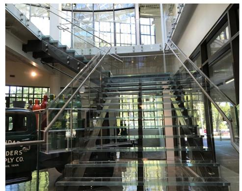
*The client wanted the illusion of invisible treads. Working on a tight schedule, Trex Commercial Products achieved the client's vision with its Point Series railing system and glass treads, for a seamless, nearly invisible look.*
