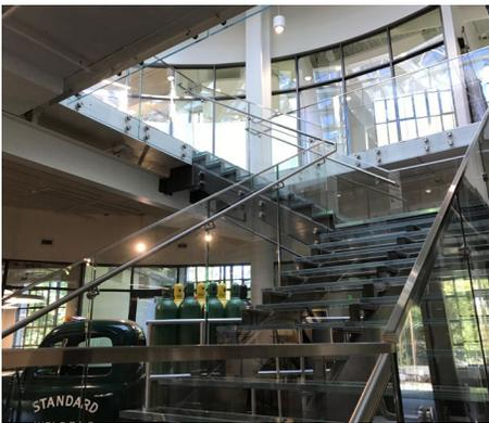
*The overlook glass was attached with a through bolt on the lower nodes and an epoxy anchor for the top.*
