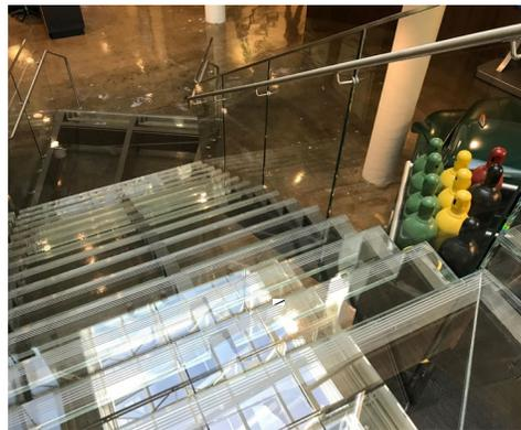
*Glass treads and risers were attached using three-inch-wide, clear VHB tape, adding to the illusion of invisibility.*
