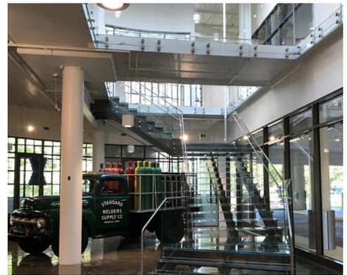
*TCP worked with the glass manufacturer and architect to come up with a tread comprised of low-iron glass with an anti-slip sandblast etch, adding functionality while maintaining the design intent.*
