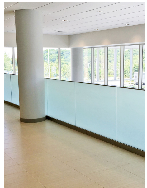
1/2" tempered laminated glass panels with a frosted interlayer create privacy without compromising the light, airy atmosphere.
