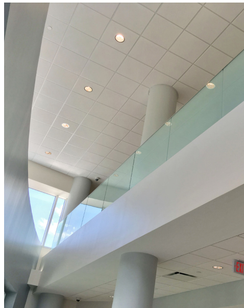
Top mounted glass railing used on the second-floor balcony overlook enhances openness and safety.
