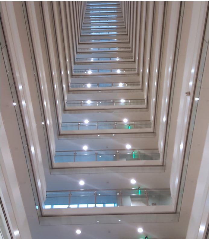
Glass balcony railing and smoke baffle utilized on multiple levels throughout the interior of the facility.
