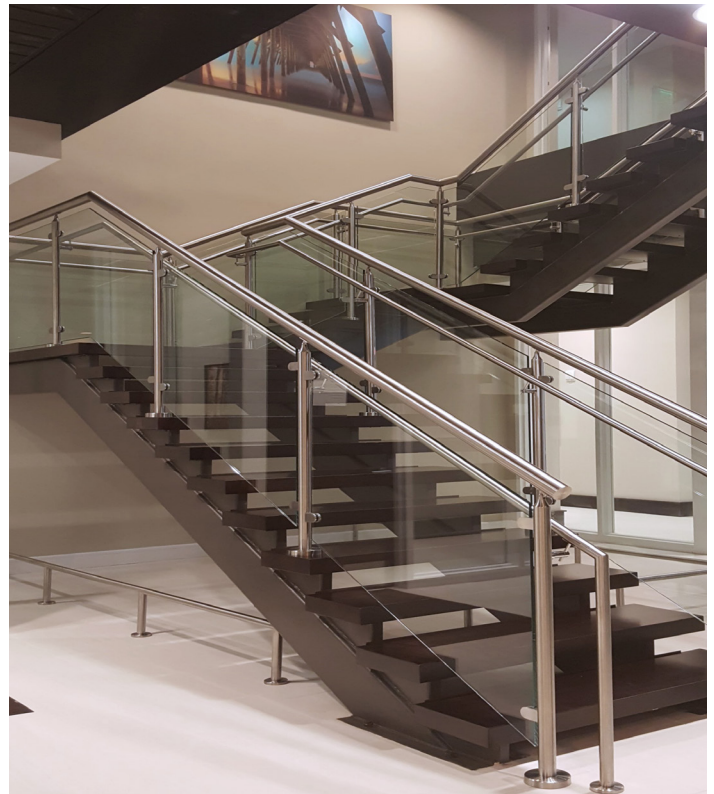
Interior Monaco stainless and glass modular railing on stairs and landings.
